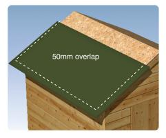
2 Cut each strip of felt so that it overhangs the edges of the roof by 50mm. Place the first strip of felt at the lowest part of the roof so that it overhangs the eaves by 50mm. Fix in position by nailing the top edge of the felt with 13mm galvanised clout nails at 500mm centres.
